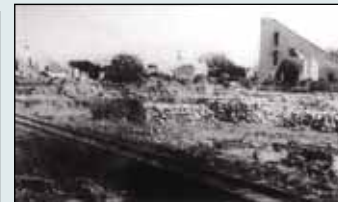
■ A railway line was laid for the project.
